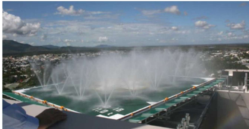
Figure II-6-8. A water-only DIFFS on a heliport with a passive fire-retarding surface
