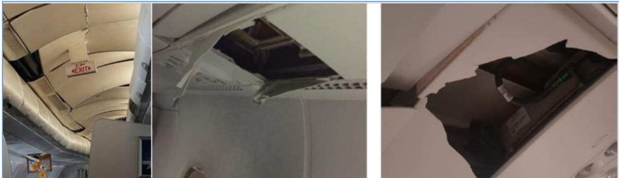
Figure 1. Examples of cabin interior damages
