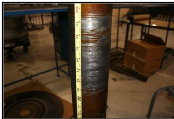
Figure 16 Example of rubbing marks (LPT shaft)
