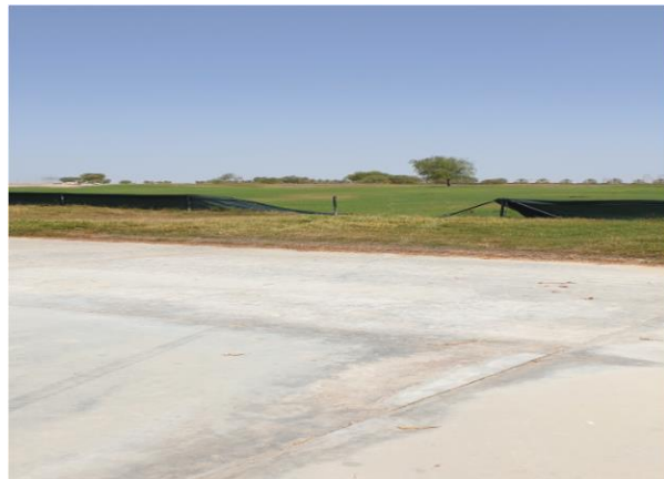
Figure 5. Damage to the fence
