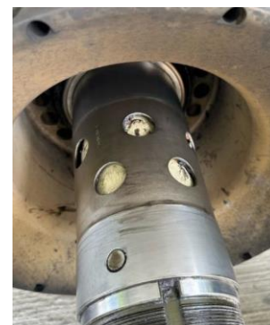
Figure 3. Overheat damage on axle sleeve
