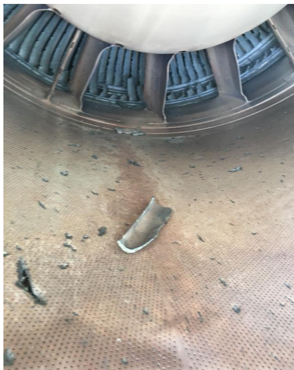
Figure 2. Damage to the No.1 engine turbine and exhaust case acoustic panel, and turbine debris
